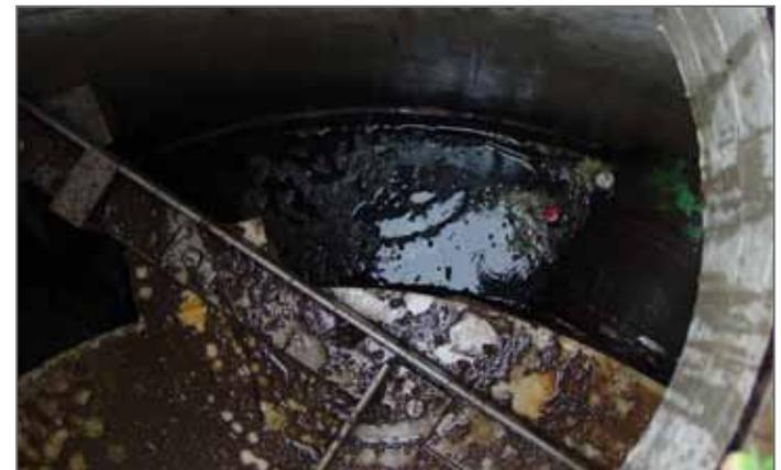
Fig. 8 View of outer annulus of floatables and oil collection zone.
