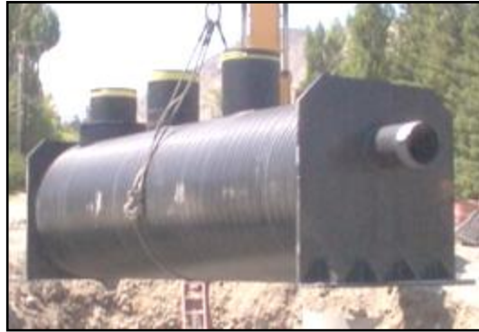
Filtration chamber of Aqua-Filter™ system being lowered into place. Access risers are visible along the top length of the chamber.
